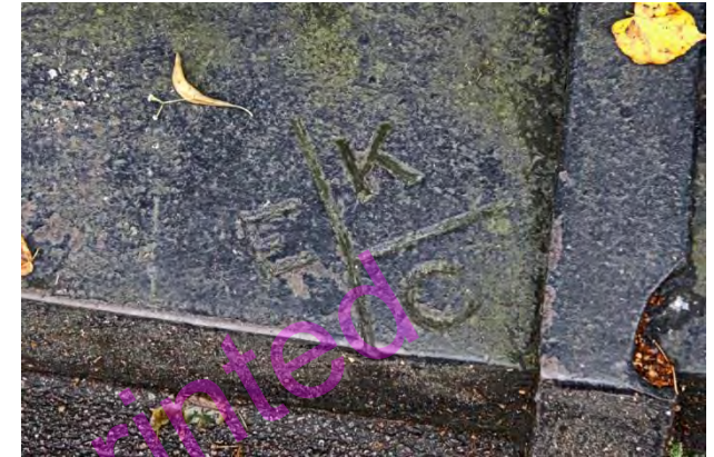
PBM 628A. Close up of the triple mark. The precision with which the trajectories are set out, and the point of convergence marked, is noteworthy.
