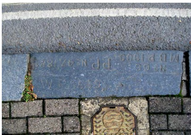
PBM 696. Kilburn Park Road, NW6. West side at junction with Rudolf Road (south side). This mark represents a horizontal boundary line, near (west) edge reads W.P. 1889. Lettering on other edge inverted. Parish of Paddington with Willesden Parish. TQ254831
