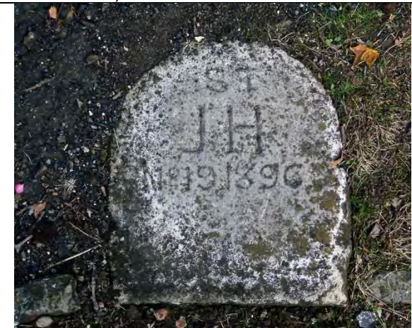
PBM 688A. Close up of the St.J.H. stone, dated 1896 and marked as No 19. This stone is located right next to large old oak tree which probably served as earlier boundary mark.
