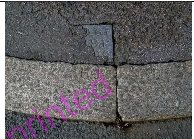
PBM 697 Kilburn Park Road, NW6. West side at junction with Rudolf Road (north side). The boundary line runs almost vertically. Visible are a Paddington Borough stone No 67. M.B.P. 1900. Below on kerb reads P.P. No 48, 1889. Feint evidence of W (for W.P.) inscribed to left. Parish of Paddington with Willesden Parish. TQ254831
