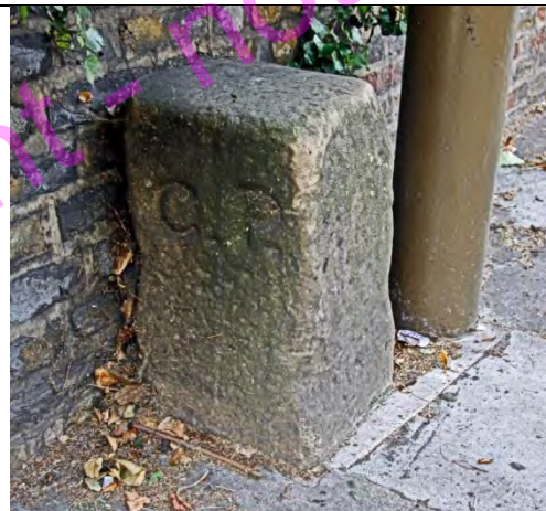
PBM 626. Charlton Park Lane SE7, North side, just west of junction with Repository Road. Stone block about 21ins high bearing initials C.P. on one side and W.P. on the other. Charlton parish with Woolwich parish. TQ425777
