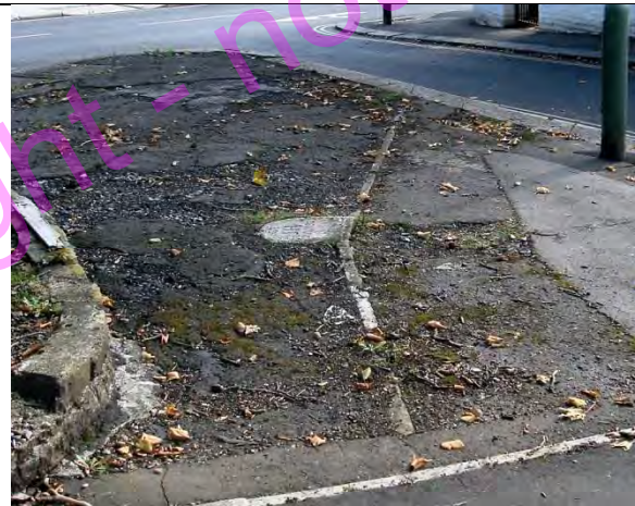
PBM 688. Platts Lane NW2. Junction with Hermitage Lane. This view looks south across the traffic island and shows stone in centre with stone-inlaid boundary line emanating from each side indicating boundary trajectory. This line is also incised in the bordering kerb stones. St John Hampstead parish with Hendon parish (and 1889-1965 Counties of London and Middlesex). TQ253862
