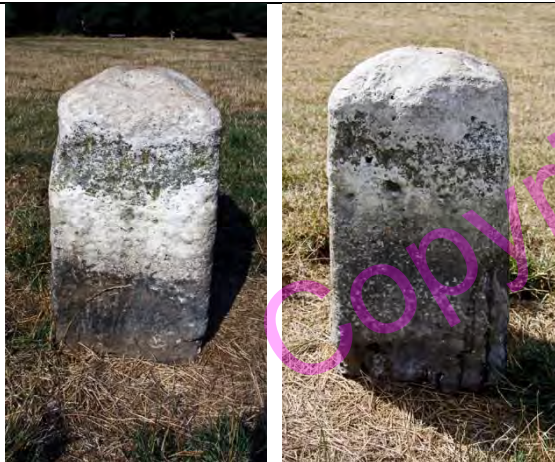
Close up views of stone working round progressively from west face to south, east and north faces. A tertiary benchmark and stud is located on top.
