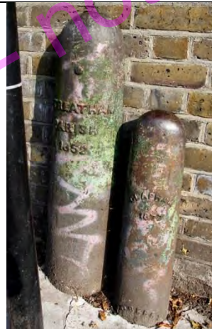
PBM 504. Cavendish Road SW12, east side, near corner with Atkins Road. A Streatham mark dated 1852 and to its right a Clapham mark dated 1877. The counter-intuitive arrangement results from it marking one end of an incursion of Streatham into Clapham parish. Clapham Parish and Streatham Parish. TQ290737
