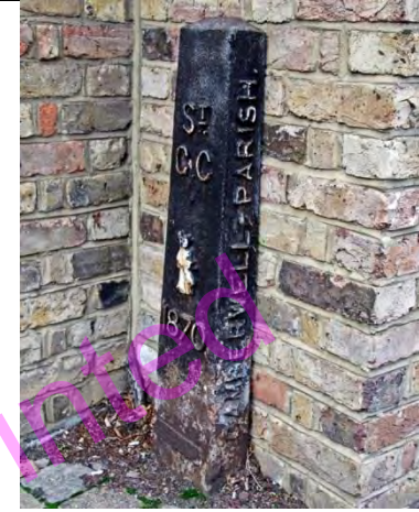
PBM 542. Sydenham Hill SE26, west side, a little south of No 133. This is a standard Camberwell 1870 mark. This mark shows a rectangular area at bottom that will be the manufacturers mark, but it is too corroded to read. Lewisham and Camberwell, and Kent and Surrey. TQ353740.
