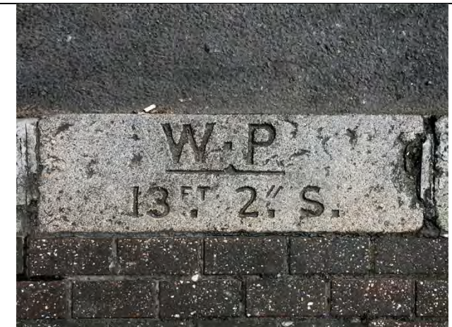
PBM 736. Kilburn Lane, W9. North side opposite east corner of Bravington Road and outside gate of No 289. A Willesden Parish mark inscribed in kerb giving distance to boundary line in centre of road. Parish of Willesden with Paddington. TQ245830
