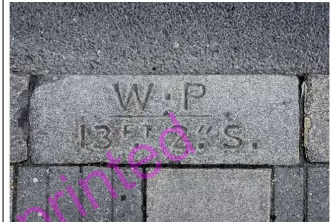
PBM 733. Kilburn Lane, W9..North side just east of corner with eastern arm of Claremont Road and opposite No 336. A Willesden Parish mark inscribed in kerb giving distance to boundary line in centre of road. Parish of Willesden with Paddington. TQ246830
