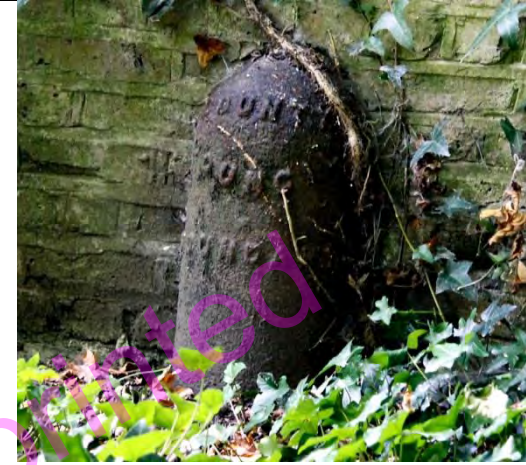
PBM 644. Parliament Hill. Alongside wall at rear of gardens along western edge, about 50yds north of Parliament Hill gate (at rear of No 93 South Hill Park). Standard LCC property mark along boundary line that follows parish boundary. St John Hampstead Parish with St Pancras Parish. TQ275860
