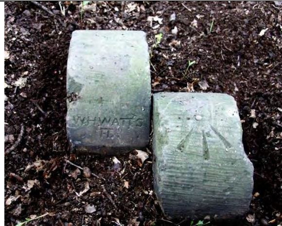
PBM 648A. Close up of edge of these stones showing benchmark (with stud) and (apparently) maker's name, the latter uncommon. Name is W.H. Watts – H.
