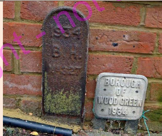
PBM 595. Curzon Road N10, west side, north of Coniston Road by No 29/31. Hornsey plate No 327. Wood Green plate in suspiciously good condition and one wonders if it is a replica. As part of the 1934 boundary adjustment this was moved south by about eight houses to cross road at right angle rather than slant. Borough of Hornsey (Clerkenwell parish detached) with Borough of Wood Green (Tottenham parish until 1894, then Wood Green parish) TQ288901.
