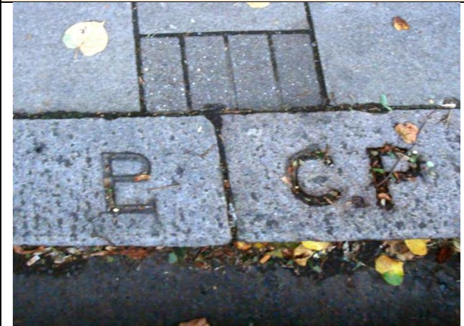
PBM 585. Burton Road SW9, north side near junction with Brief Street. An excellent example of a kerb marker, a type unusual in south London. On left is Lambeth monogram, and on right Camberwell initials.
