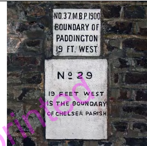
PBM 715. Kilburn Lane, W10. East side at junction with Banister Road in wall of No 104. Boundary line runs along centre of road, 19ft away according to inscription. Top mark is Paddington Borough 1900 No 37. Bottom is Chelsea Parish No 29 (absorbed by Paddington in 1900 – unusual to leave older mark). Parish of Chelsea (detached) with Parish of Willesden. TQ238828.
