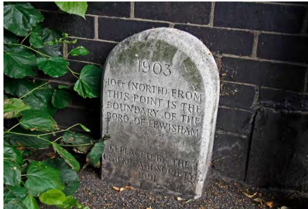
PBM 603. Blackheath Grove SE3. South side at base of wall of railway. A Lewisham Borough tombstone type mark, though actually claiming to be a 1991 replacement. Mark relates to 1903 border alterations. However the boundary was the wall behind this stone and not 10ft in front, so it appears an error has been made. Lewisham Borough (Lewisham Parish) with Greenwich Borough (Charlton Parish). TQ396760
