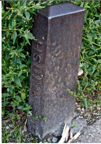
PBM 528. Gipsy Hill SE19, east side at extreme north end. This is of same style as PBM 531, but with its 'blind' side facing the road. The rear cannot easily be read but is probably dated 1874 like its neighbour. Parish name 'Camberwell Parish' appears along either narrow edge (in this case partly buried). Lambeth parish and Camberwell parish. TQ331716
