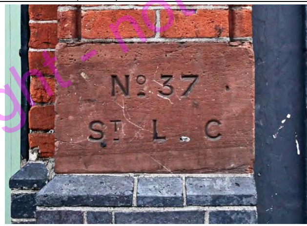
PBM 717. Harrow Road W9, north side east of Bravington Road. On pilaster separating 570 and 572. This seems to be part of former church property and presumably dates to that building in 1883-4. A nice survivor from St Luke Chelsea. Parish of Chelsea (detached) with Parish of Paddington. TQ245823.
