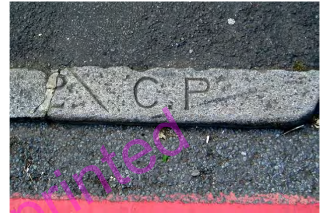
PBM624. Camberwell Station Road, SE13. West side on corner with Camberwell New Road. This is a stone common to both parishes, Lambeth mark on left, Camberwell on right and oblique line showing trajectory of boundary. The stone appears correctly located, but has evidently been disturbed at some time with some loss on left side. Camberwell Parish with Lambeth parish. TQ323768
