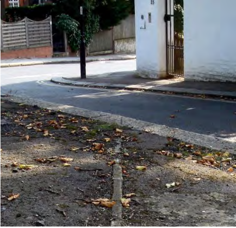
PBM 688B. This image shows the boundary line and incised kerbstone looking south. The boundary turned right to run with the boundary wall (the corner visible here) along Platts Lane.
