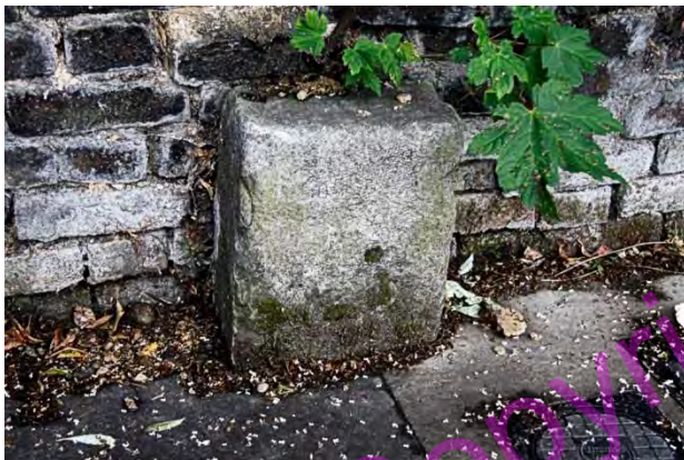
PBM 629. Shooter's Hill Road SE18, south side, outside No 122 (opposite garage). This stone is so badly weathered as to be unreadable. It probably indicates division between Charlton and Greenwich parishes as Kidbrooke ran with wall behind. Charlton parish with Kidbrooke parish and Greenwich parish. TQ409771
