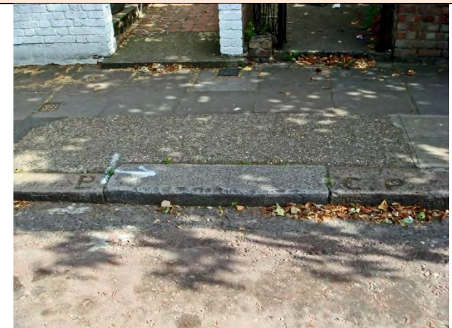
PBM 623. Knatchbull Road SE5. South side, just east of County Grove, at speed hump (opposite PBM 621). The centre stone is obviously more recent than the others and examination of maps suggests the Camberwell stone has been displaced to the right by its insertion.
