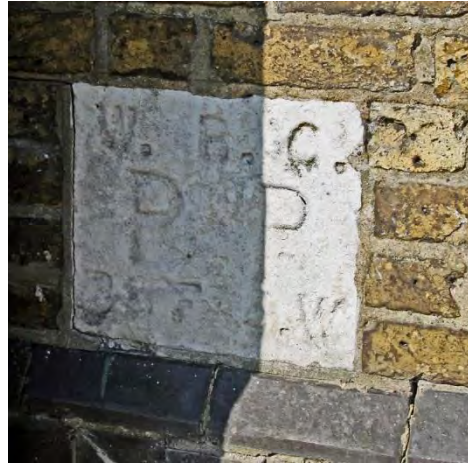
PBM 658. Upper Wickham Lane, DA16, east side by Lodge Hill. The distance at bottom of this wall-mounted stone indicates the location of the boundary line along road centre. The stone is in Plumstead and the letters mean Woolwich Borough Council (dating it after 1900), Plumstead Parish. It is possible the Woolwich marks are a later addition to a much earlier stone though. Plumstead Parish and East Wickham Parish (and from 1889-1965 County of London with Kent). TQ467770
