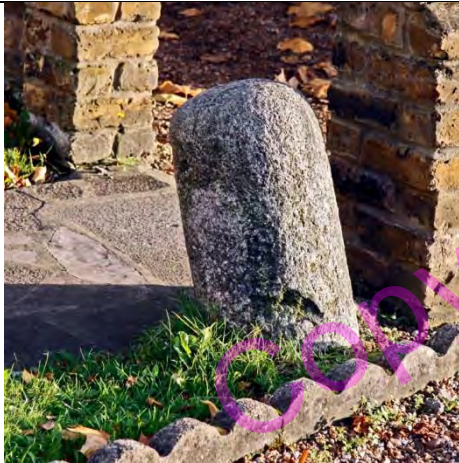
PBM 565. Kent House Road BR3, east side at corner of Barnmead Road (in garden). This weathered stone is unreadable, although odd letters can be made out. It is exactly on a boundary line though old maps do not note it as a boundary stone. Further investigation required. Beckenham parish and Penge Parish (and Kent [later County of London] with Surrey). TQ359699.
