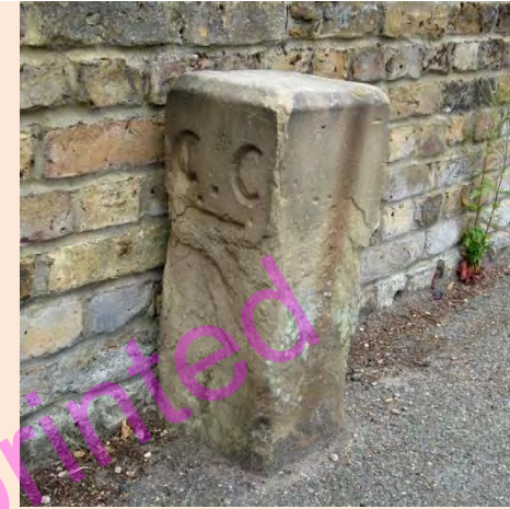
PBM 621A. East face of the same stone. This face shows C.C. - L. This face is also spalled, where the 'L' would appear.
