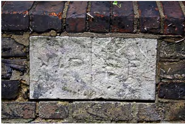
PBM 627. Herbert Road SE18, north side, just west of junction with Llanover Road. Stone tablet about 9ins high bearing initials W.P. on left, then a vertical boundary line and P.P. on the right. Woolwich parish with Plumstead parish. TQ432772
