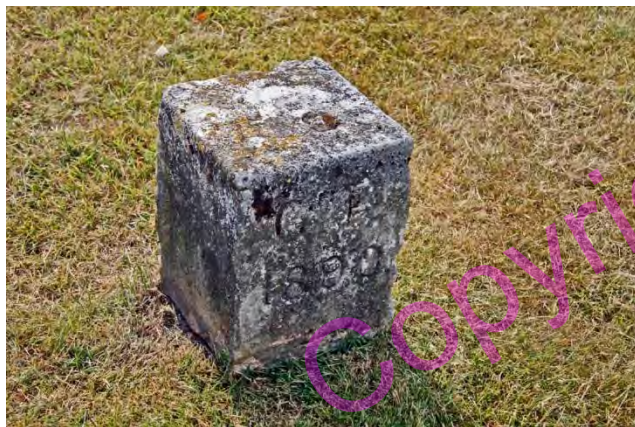
PBM 611. The Paragon SE3. North side, opposite No 8. A Greenwich rectangular section stone column dated 1890. This appears to have been left in position after 1903 boundary alterations. There is a benchmark on reverse. Greenwich Parish with Lewisham parish. TQ400763
