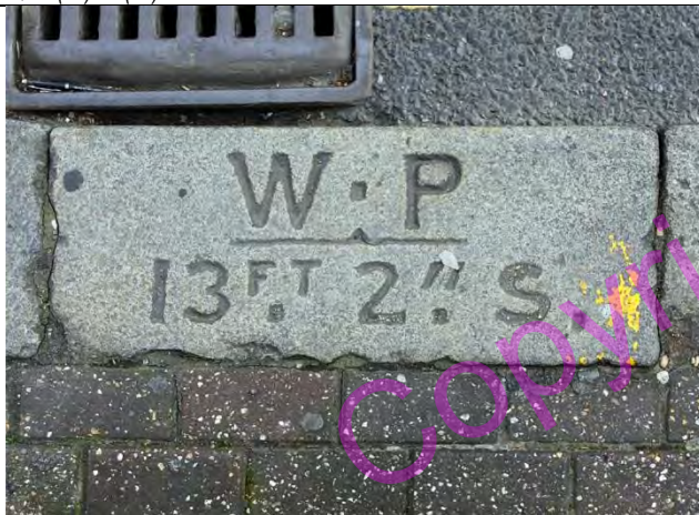
PBM 734. Kilburn Lane, W9. North side just west of corner with eastern arm of Claremont Road and opposite No 334. A Willesden Parish mark inscribed in kerb giving distance to boundary line in centre of road. Parish of Willesden with Paddington. TQ246830
