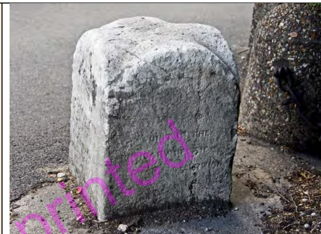
PBM 599. Blackheath Hill SE10. North side, at former junction with Point Hill. Opposite No 134. Square section stone block with symmetrical arched top. Heavily weathered but lettering reveals Borough of Greenwich stone referring to boundary nearby (direction change centre of junction). Two faces are clearly lettered. Borough (parish) of Greenwich with Borough (parish) of Lewisham. TQ384767
