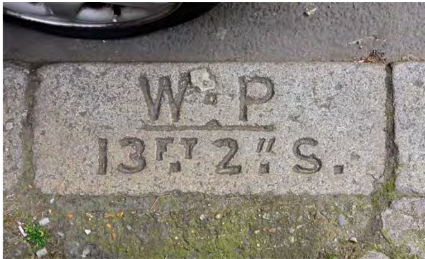
PBM 737. Kilburn Lane, W9. North side opposite west corner of Bravington Road and outside p/w of No 283/5. A Willesden Parish mark inscribed in kerb giving distance to boundary line in centre of road. Parish of Willesden with Paddington. TQ245830
