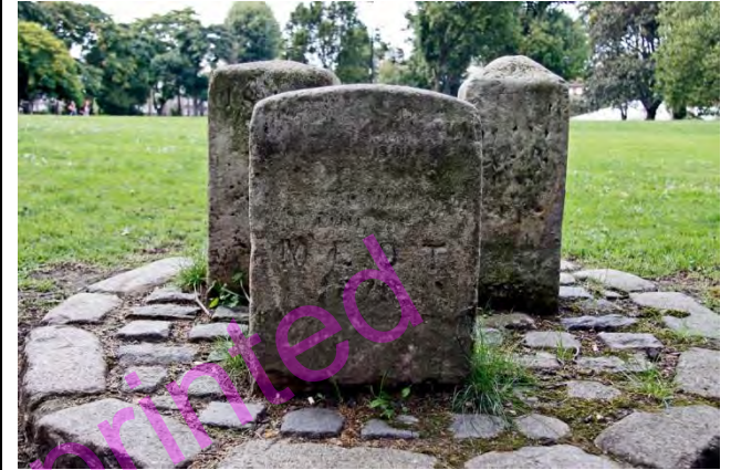
PBM 667A. View faces north. The nearest stone appears to read '...The Boundary Line of M.E.O.T 1876'. There is lettering in front almost certainly giving the distance of the boundary from the face of the stone. Maps show a pair of stones several feet from boundary (which had run through Devonshire Street railway goods yard where correctly located stones would have been in the way). Meath Gardens had once been Victoria Park cemetery.
