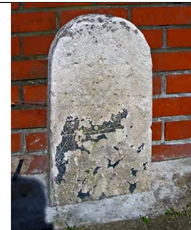
PBM 706. Junction of Woodyates and Guibal Roads, SE12, east side. This appears to be a mark of identical style to PBM 705 and probably relates to boundary direction change in centre of road about 20ft away (boundary ran through No 173, to south). Borough of Lewisham (Lee Parish) with Borough of Woolwich (Eltham Parish). TQ405736
