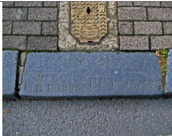
PBM 696A This is the other (east) edge of previous mark showing the Paddington edge. Left hand side reads No 66. M.B.P 1900 (for the new Borough). RHS reads PP No 47, 1889. It appears this stone originally divided parishes along long edge, and Paddington Borough information added later. Parish of Paddington with Willesden Parish. TQ254831
