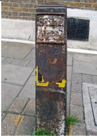
PBM 668A. This shows the face of the post, marked St.M.I. 1838 in the tablet. This very old post has all the characteristics of a boundary mark, and lies on the boundary, but it is very unusual in being located along the vulnerable pavement edge. It is shown on the 1896 OS 1:1056 map marked as a boundary post and would not have been shown thus if it were regarded as a bollard.
