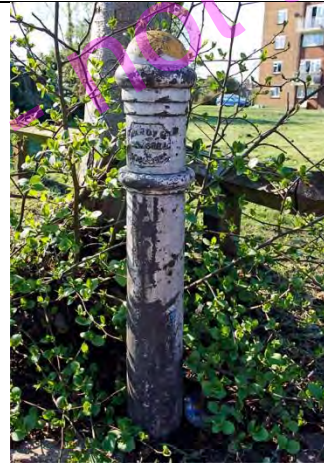
PBM 566. Kent House Lane BR3, west side where it becomes Bell Green Lane at brow of hill. This is a dome topped cylindrical metal post buried in bush, exactly on boundary deviation and shown on old maps. No parish name (lettering at top is maker). Last survivor of row of posts marking boundary line on Lewisham side. Beckenham parish and Lewisham Parish (and later County of London with Kent). TQ364712..
