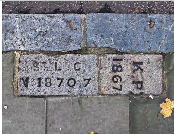
PBM 713. Southern Row W10. South side, in pavement 40ft west of Bosworth Street building line. Surprising survivors in redeveloped street, A Chelsea mark on left with number and Kensington mark on right. Boundary crossed road here. Parish of Chelsea (detached) with Parish of Kensington. TQ243821.
