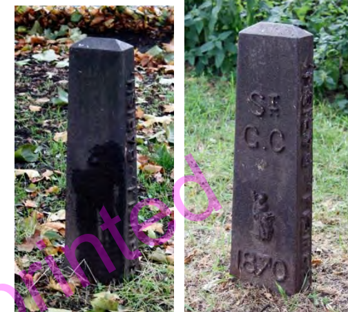
PBM 588. Cormont Road SE5, east side behind railings about 20 feet behind PBM 587 (in Myatts Fields in front of tennis court). This marked change in trajectory of the boundary. It seems dogs find these posts useful even if most people do not know what they are and the Myatts Fields website ignores them. Dated 1870. Lambeth Parish and Camberwell Parish TQ317767.
