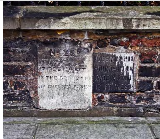
PBM 714. Kilburn Lane, W10. East side near south end outside No 36, near junction with Chamberlayne Road. Boundary line runs along centre of road, 17ft away according to inscription. RH mark is Paddington Borough 1900 No 36. LH is Chelsea Parish No 28B. Paddington absorbed this part of Chelsea (det) in 1900. Parish of Chelsea (detached) with Parish of Willesden. TQ238827.
