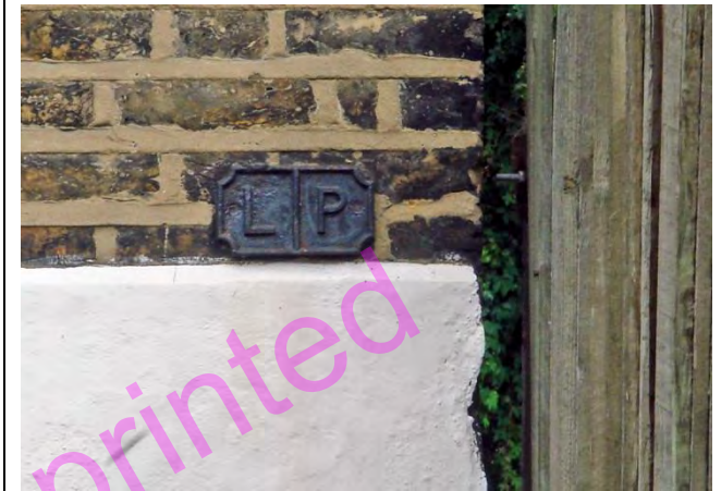
PBM 604. Collins Street SE3. East end. Rectangular metal plate with notched corners bearing initials LP. (Lewisham Parish). Significance of vertical line not apparent, but actual boundary understood to be at corner of brickwork on right.. Lewisham parish with Lee Parish. TQ395760.
