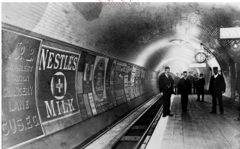
Cross-track advertising at this just-opened Central London Railway tube station clearly dominates. The assortment of sizes suggests a desire to accommodate advertisers as much as possible.
